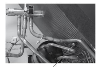
Electronic expansion valve coil
