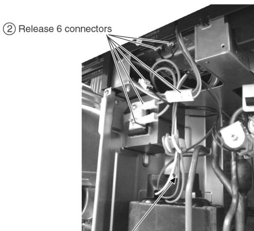
① Remove the screw then release the 3 connetors inside
